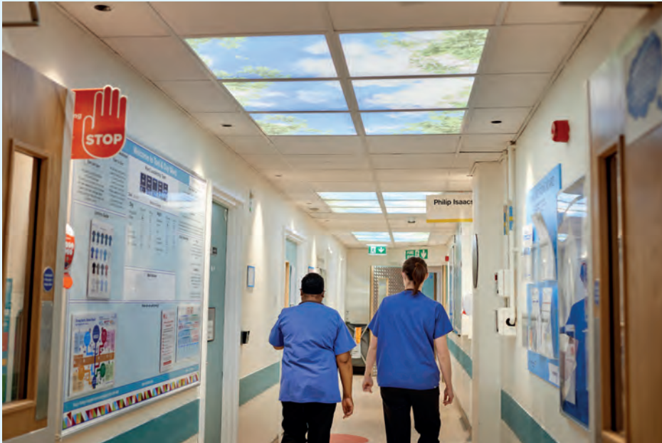
Above: Artificial skylights in Majors
