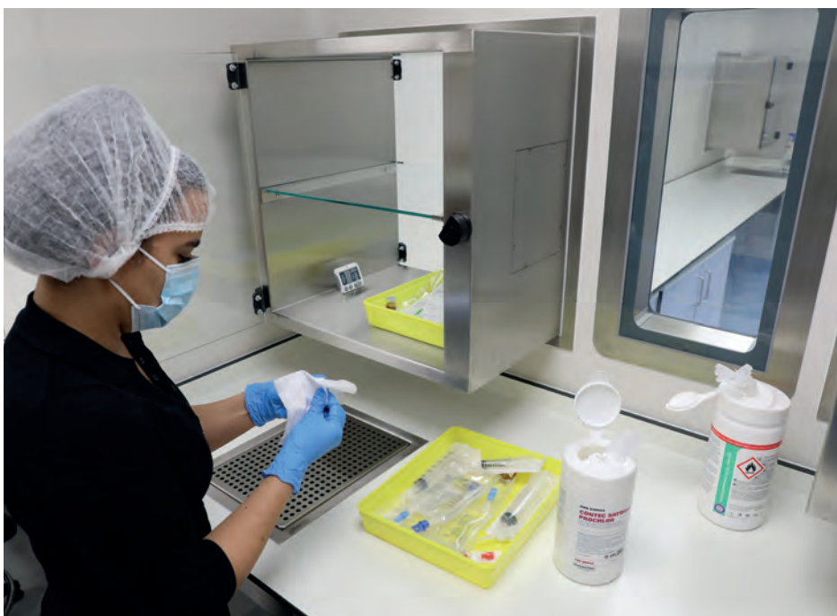
Above: Medicines are passed between rooms through sterile, air lock style hatches
